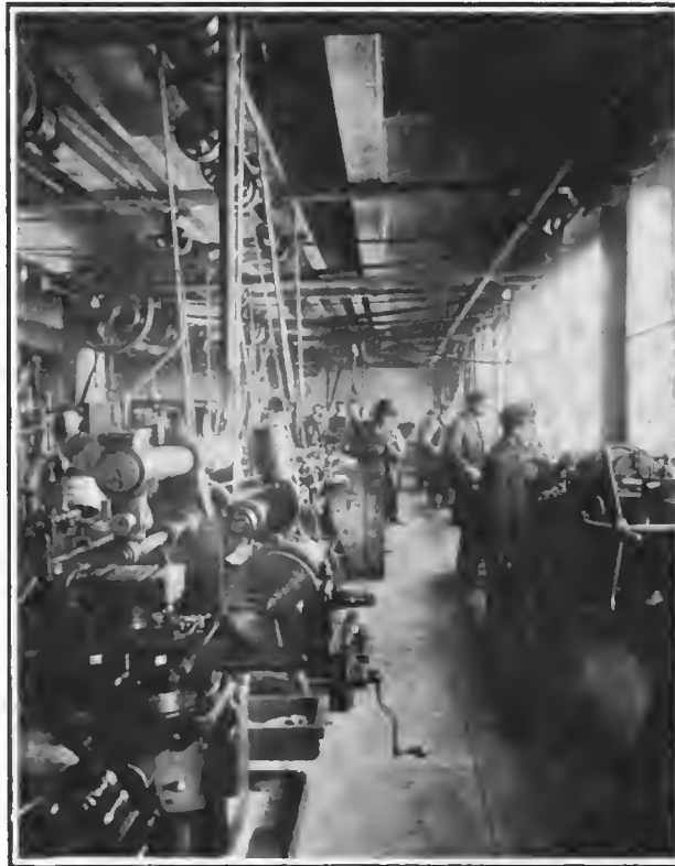
ONE END OF MACHINE SHOP IN REPAIR DEPARTMENT.
